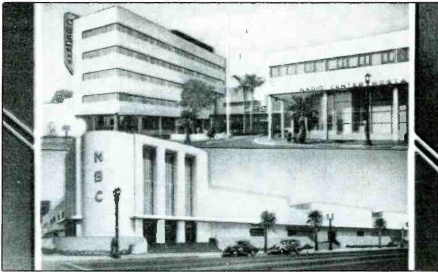
The WJPF studios were small town, mini-version of the type of architecture being used by the network headquarters in Hollywood, rounded corners and all. Compare it with the NBC studios at the bottom of this view.
